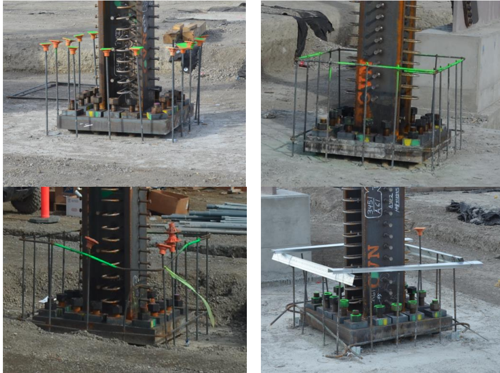
Figure 14: Different Means for Capping Rebar for Safety (© 2014 Iris D. Tommelein. All Rights Reserved.)
