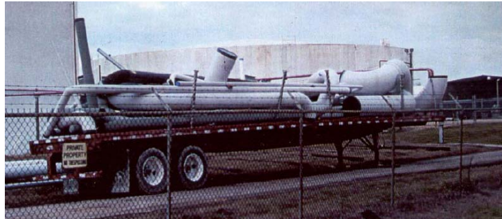
Figure 2: Staging of Pipe Spools (© 1995 Iris D. Tommelein. All Rights Reserved.)
