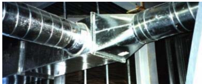
Figure 4: Tapered fitting connecting round to rectangular duct
