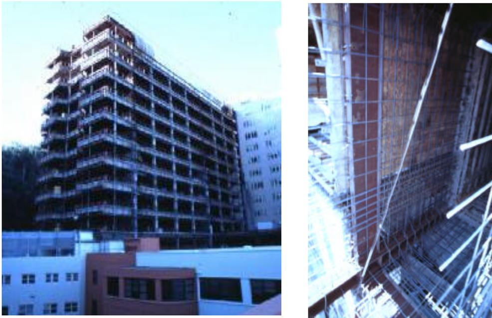
Figure 1.7. A view of 18-story hospital and close-up of a shear wall
