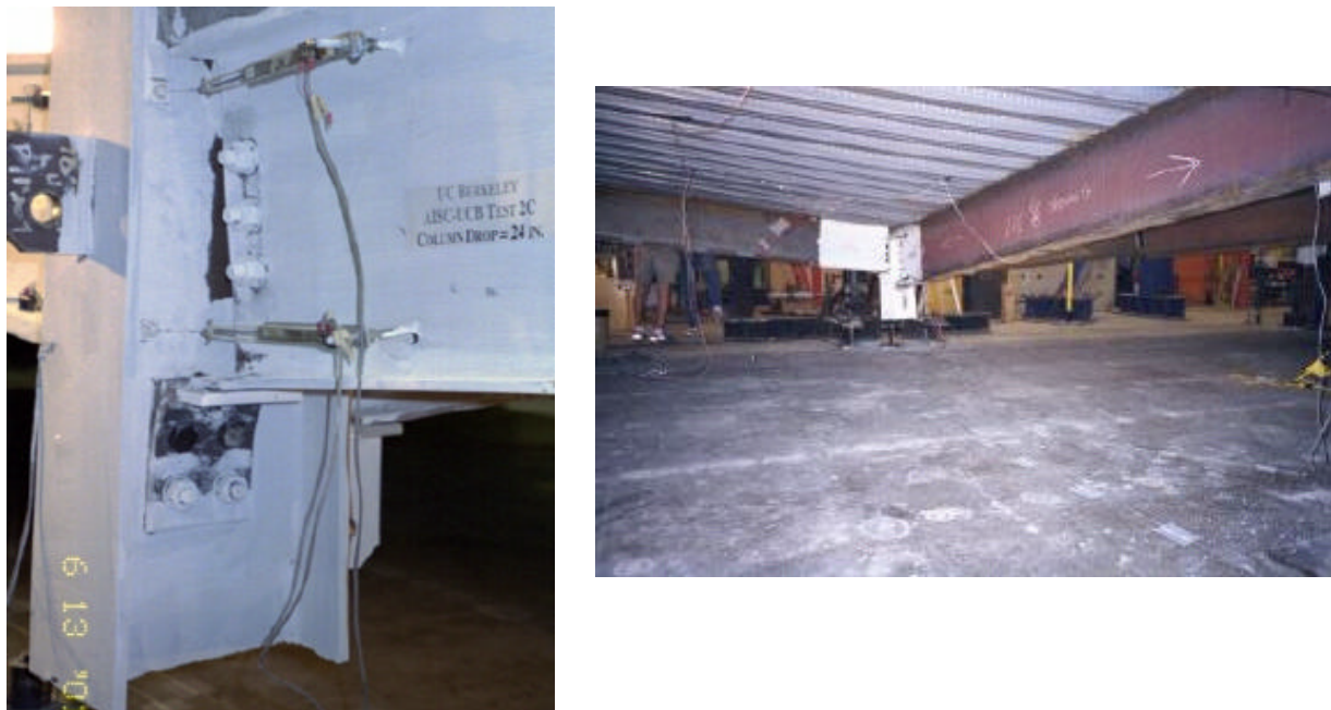
Figure 3.7. The Two Bolts on The Seat Angle Were no Longer Present
