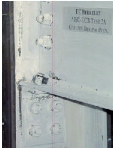
Figure 3.3. Failure of the Two Bolts on the Seat Angle
