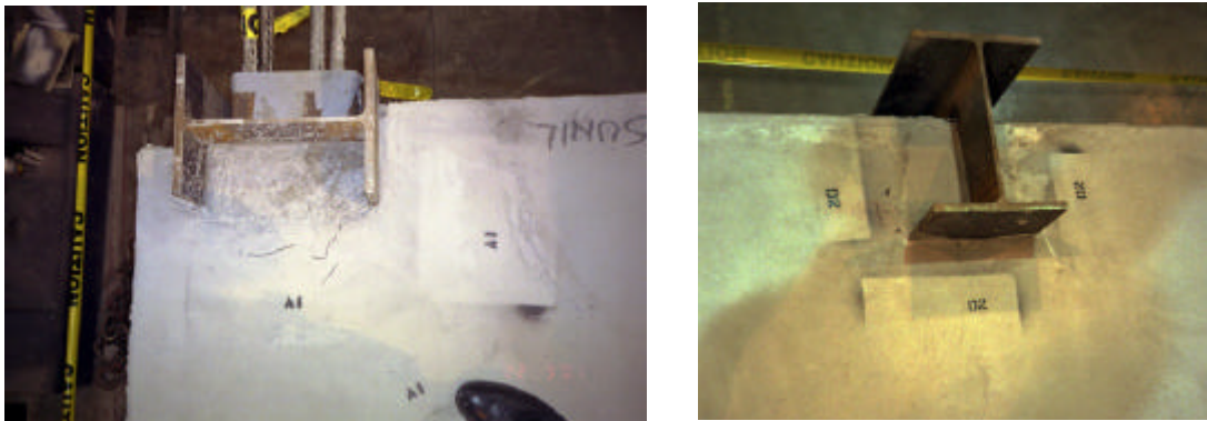
Figure 2.7 Close-up View of Slab in the Column Areas
