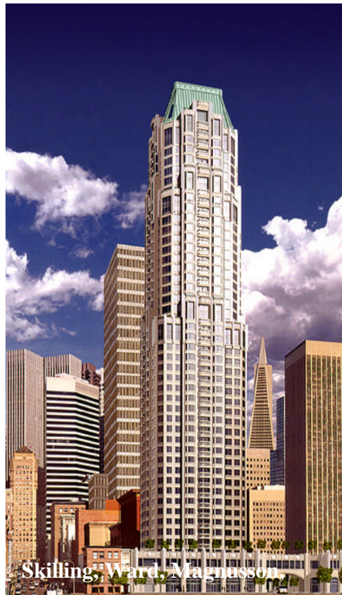
Figure 2. The 51-story building with dual steel plate shear wall system (Designed by Skilling, Ward, Magnusson, Barkshire of Seattle. Rendering courtesy of SWMB)
