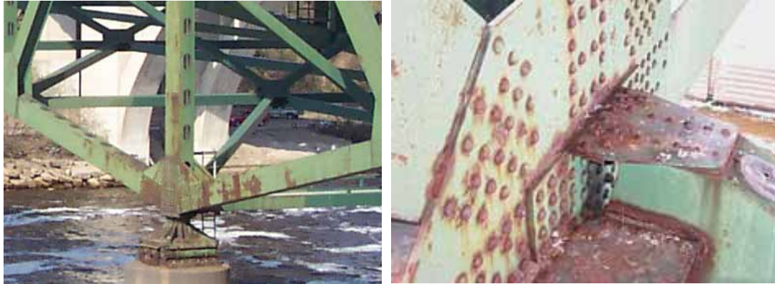
a) corrosion of roller bearing
