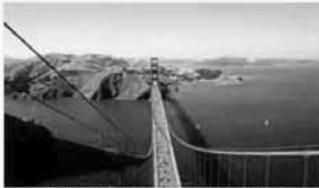
Golden Gate Bridge, Photo by A. Astaneh
